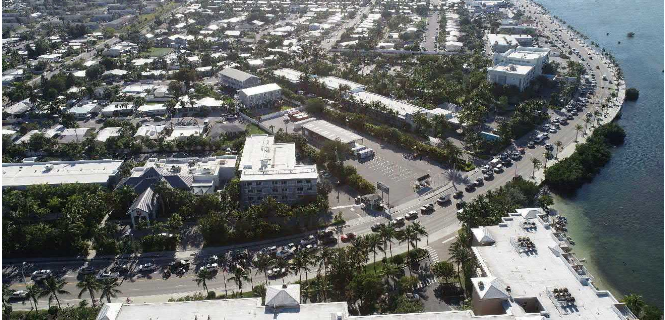
Figure 6-2: EB left-turn queues from the US 1/Roosevelt Blvd Intersection
